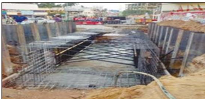
Figure 2: Gudiakhal Sluice in Puri, 2025
