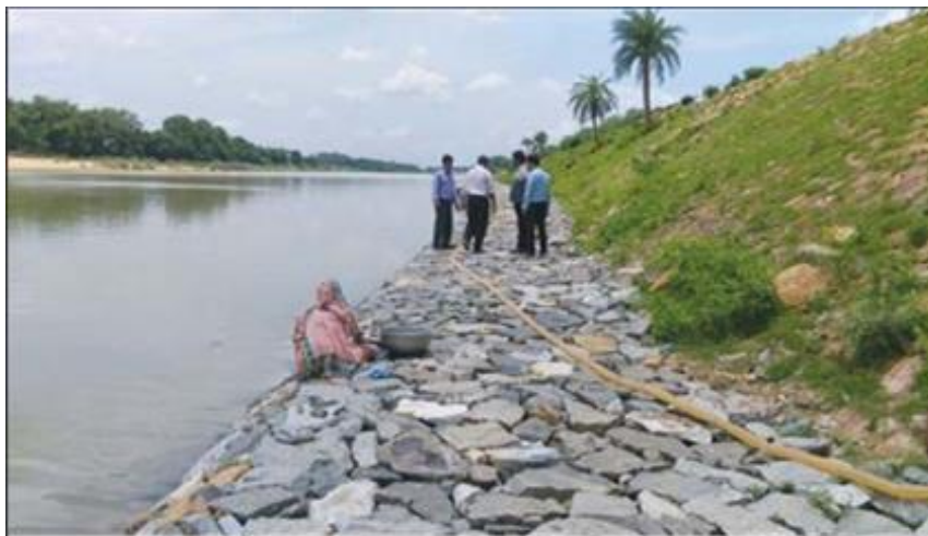
Figure 1: Slope Protection on Mahanadi Embankment at Padmabati, 2024
